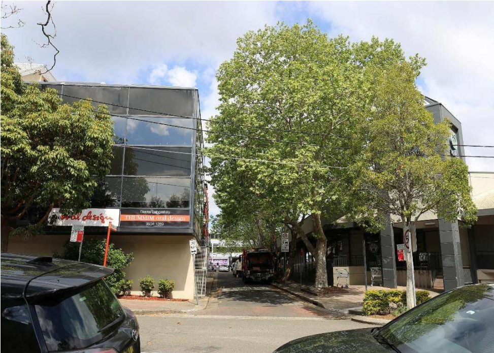
Image 1 -View from Grosvenor Street, looking South down Waters Lane
