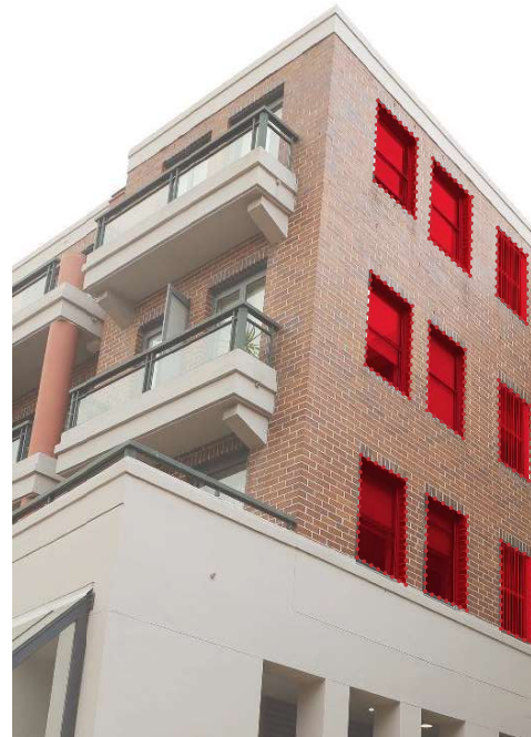
Photo of Existing
