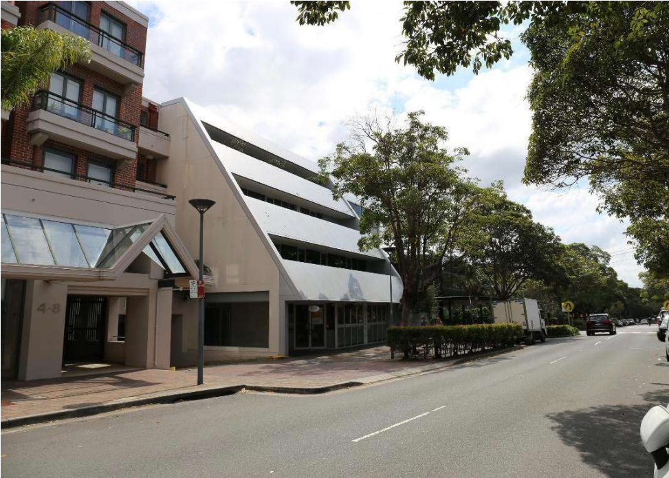
Image 1 - View looking North along Waters Road.
